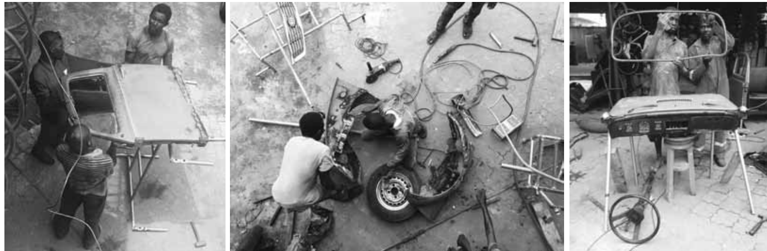
Process of build.
